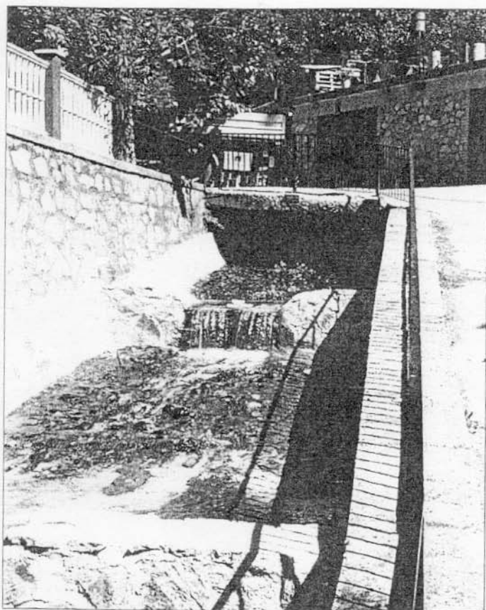
Figure 15.11 The Lagarelle Torrent canalized and partly covered where it crosses the Piedipaterno Village. The canalized cross section is too small to contain flash floods and debris flows
